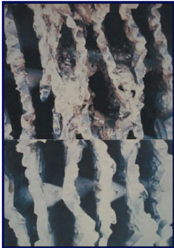
4A Composite photograph. Top--Fouled cooling tower fill. Fouling in this case was a variety of microbes and the slime they produced. Bottom--Clean cooling tower fill.
